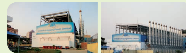
United Ashuganj Power Limited
